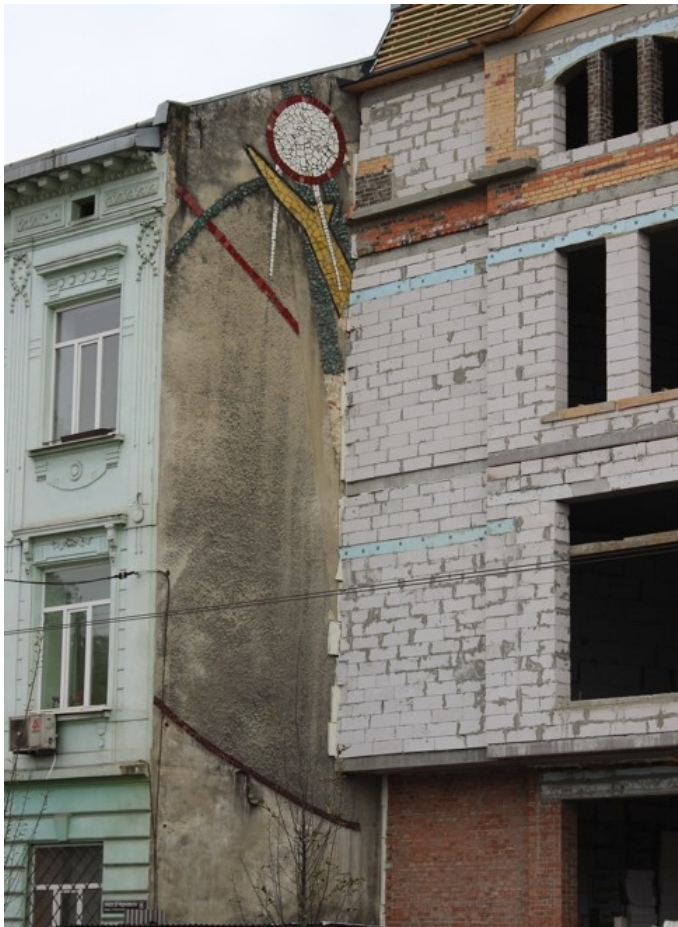
Fig. 5 – Building in Čornovil prospect 39, Lviv 2017. Source: courtesy of Olga Martynchuk.
